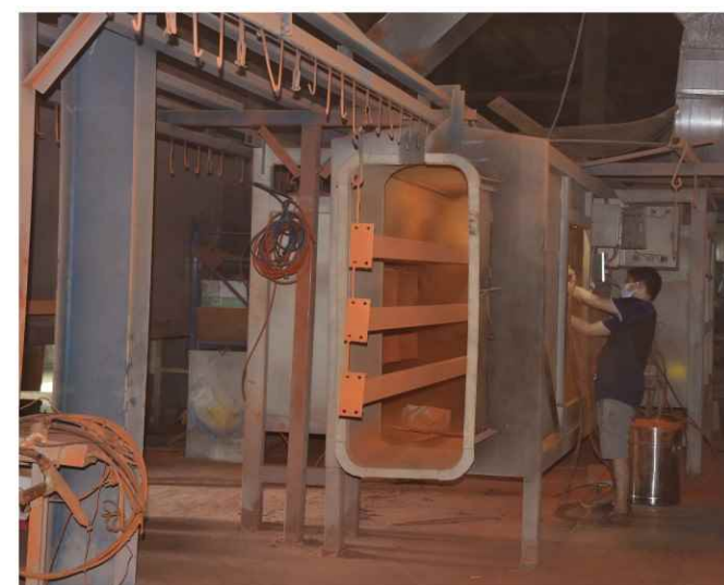
Painting line 喷涂线
