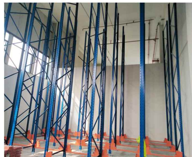
Installation of radio-shuttle racking 穿梭式货架安装
