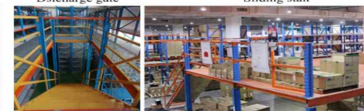
Mezzanine rack basic structure 阁楼式货架基本结构
