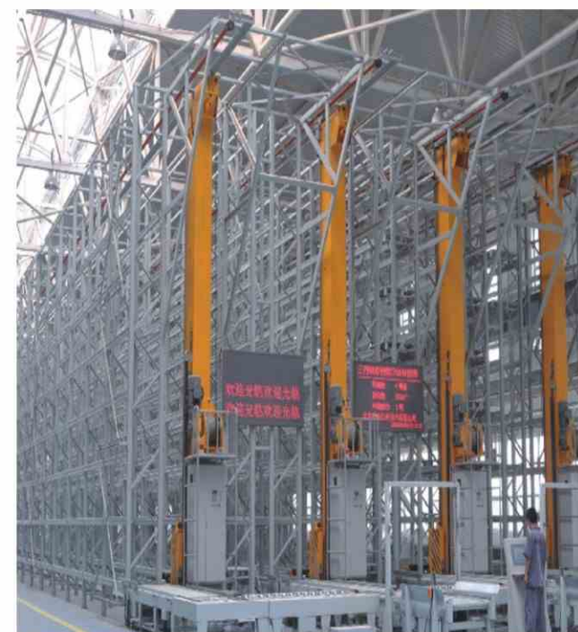
Automated warehouse ASRS system 自动化立体仓库ASRS系统
