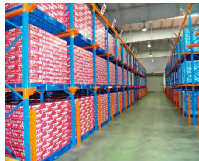
Drive-in rack project 驶入式货架案例
