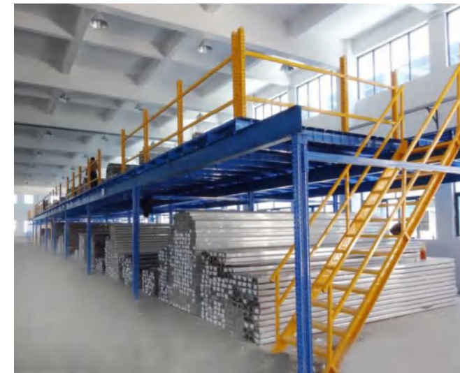
Mezzanine floor project 钢平台案例
