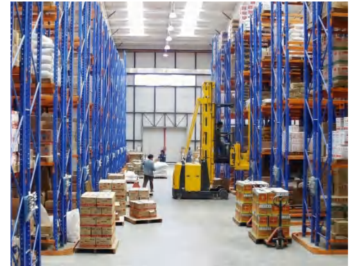
VNA rack project 窄巷式货架案例
