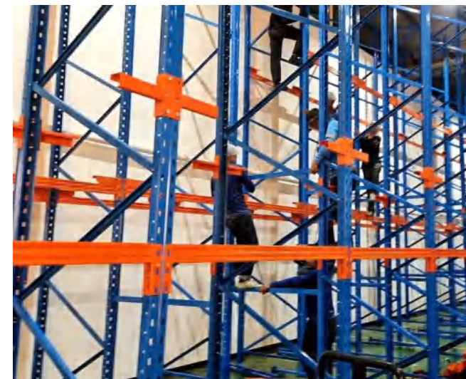
Drive-in rack project 驶入式货架案例
